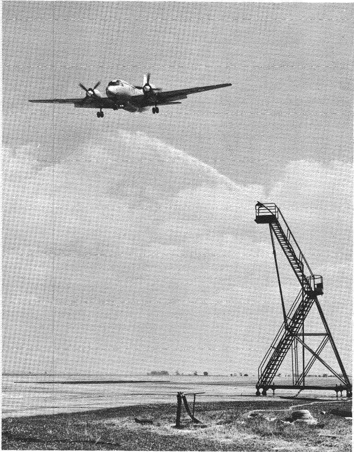
Fig 4. Simulated barrier used for Varsity trials
