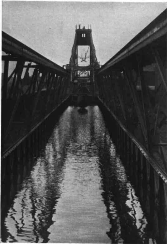
Looking towards the winch house.
