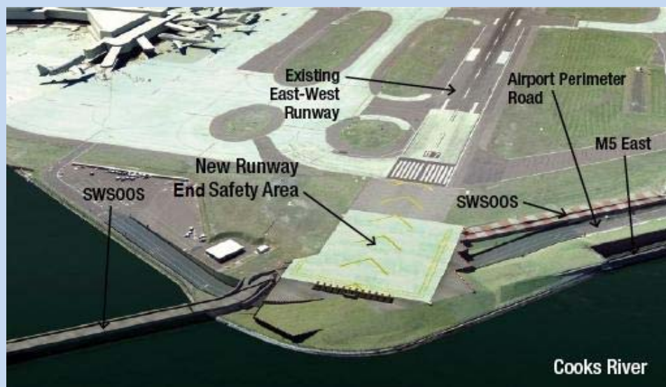
Figure 12: Sydney Airport cross-runway RESA extension, runway 07 end
