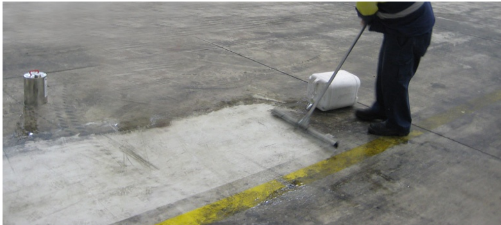
Figure 6: Chemical removal of rubber deposits from a runway
