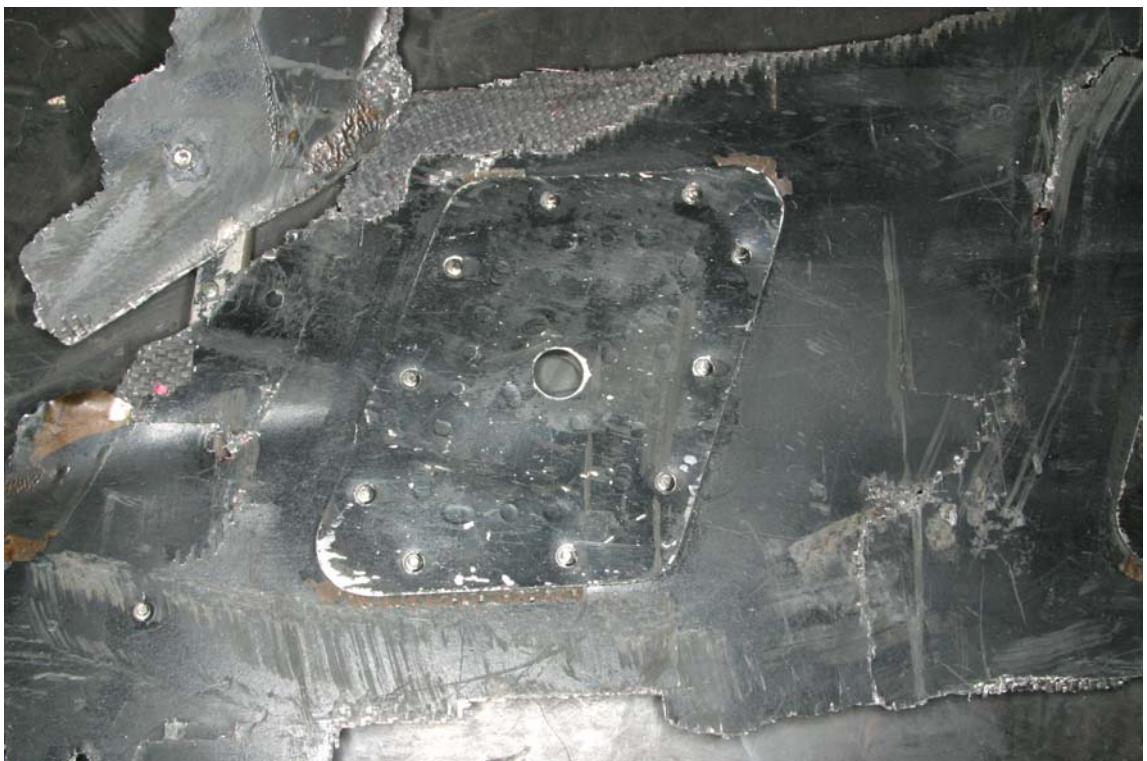
Figure 14. External drive fairing panel showing the reinforcing plate associated with the bolt towers. Compare the appearance of this plate with the impact witness mark found on one of the thrust reverser blocker doors (figures 7 & 8).
