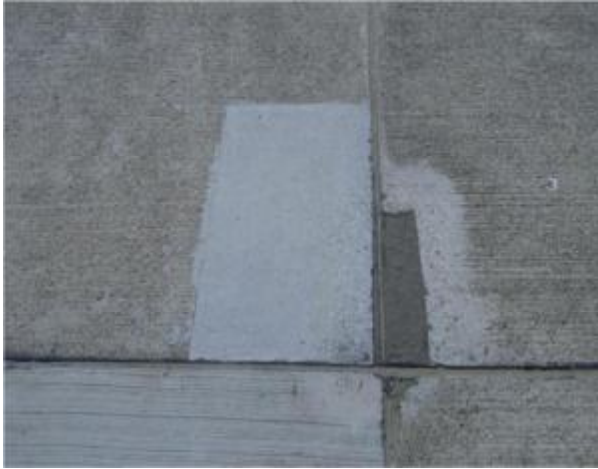
Example of "Good" Concrete Repair
