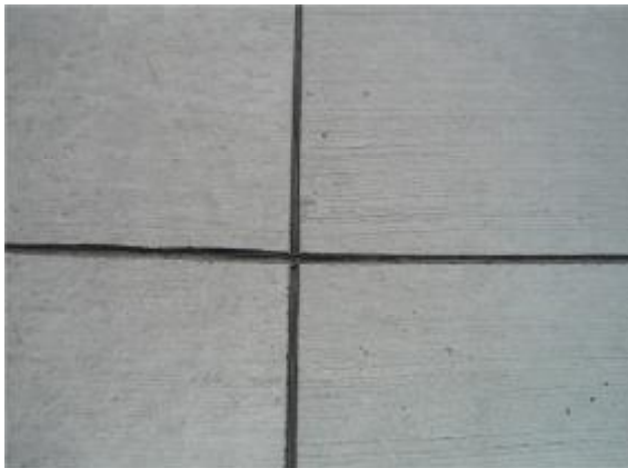
Example of "Good" Concrete Joint Sealing
