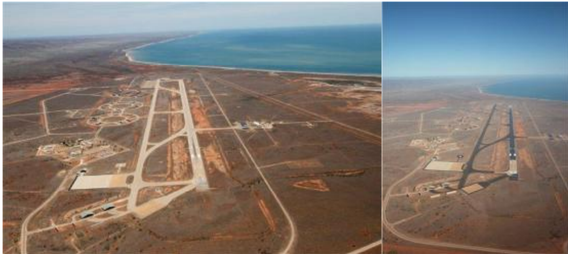
RAAF Base Learmonth – Before and After PME Surface Treatment in November 2011
