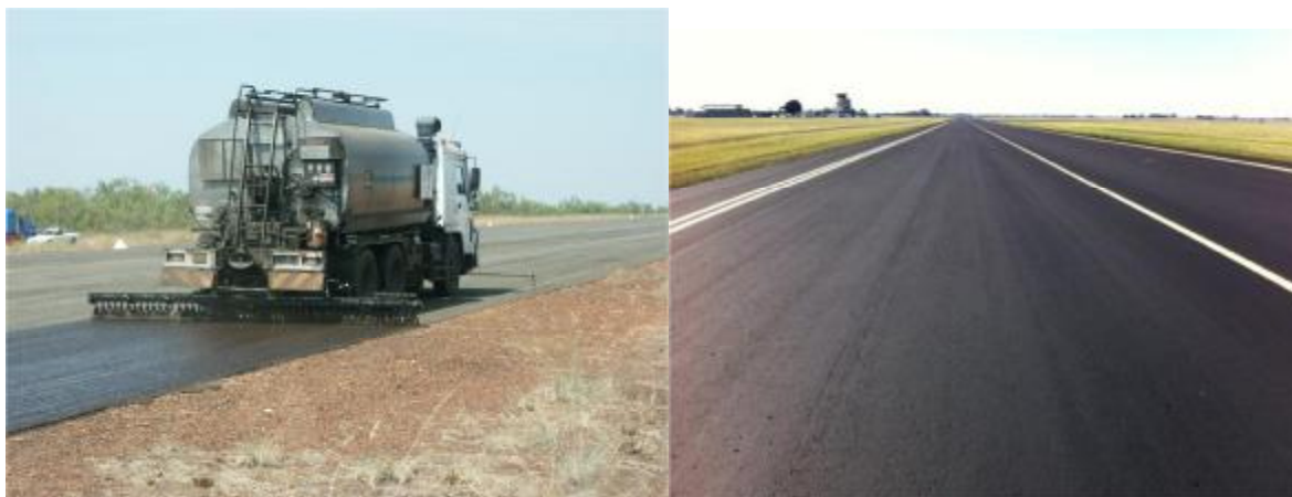
PME Application to Chip Seal Surface (Mount Bunday - August 2012) - Aged Asphalt - Pavement Treated with PME
