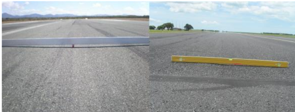
Examples of Deformation in an Aircraft Wheel Path
