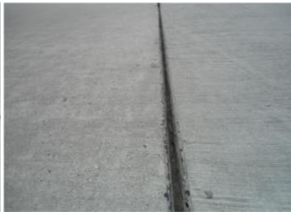
Chamfered Concrete Joint
