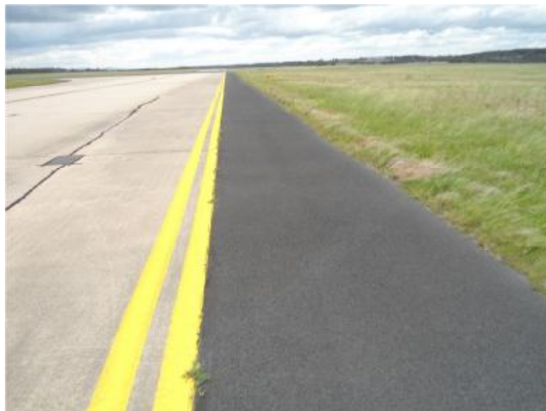
Asphalt Surfaced Taxiway Shoulder
