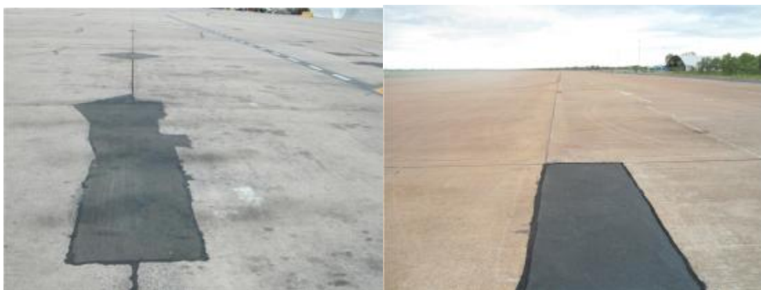
Examples of Hot Asphalt Joint and Corner Spall Repairs in Concrete Pavements
