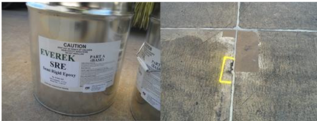
SRE(S) Repairs in Concrete Pavements
