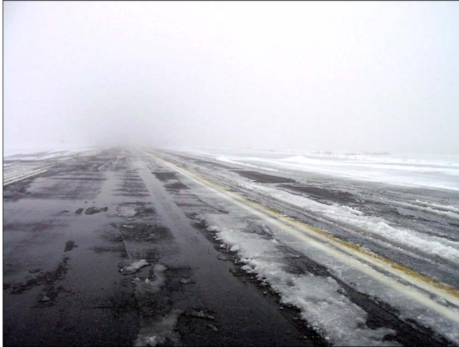
Figure 3.13: Non-Uniform Surface Conditions on a Runway in Canada
