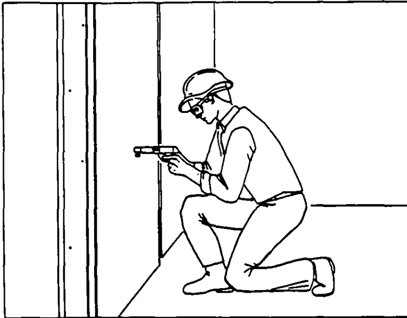
Figure 10. Installation of laminates using powder-driven fastener.
