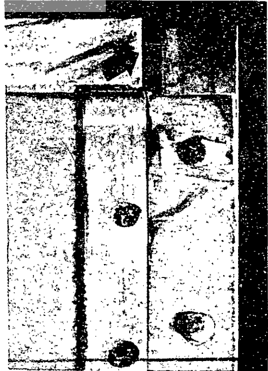
No. 35—SHORT TOP. Minor. (Extending more than \frac{1}{8} " inside cleat at both ends.)
