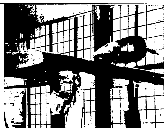
N. A. O. A. cowled nacelle, not faired into wing.
