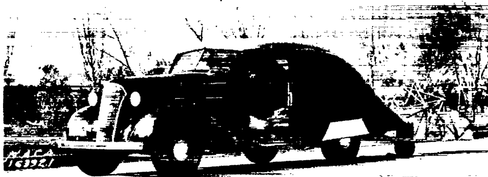
Figure 1.- Towcar with towcart attached. Castered wheel about to strike bump.
