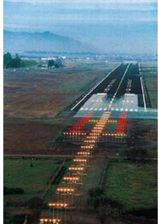
Siemens AFL photo
